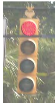
4-Section Signal Head T Configuration, In-line Configuration
