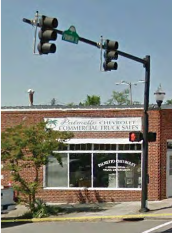
Single Mast Arm, Powder-coated, Non- decorative, no luminaire, Powder-coated pedestrian heads and signal heads
