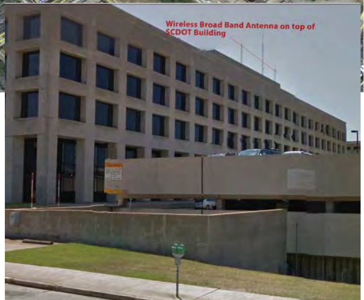
Figure 3-4 Wireless Broad Band Communications Link btwn SCDOT building & signal @ Meeting Street/Sunset Blvd.,
