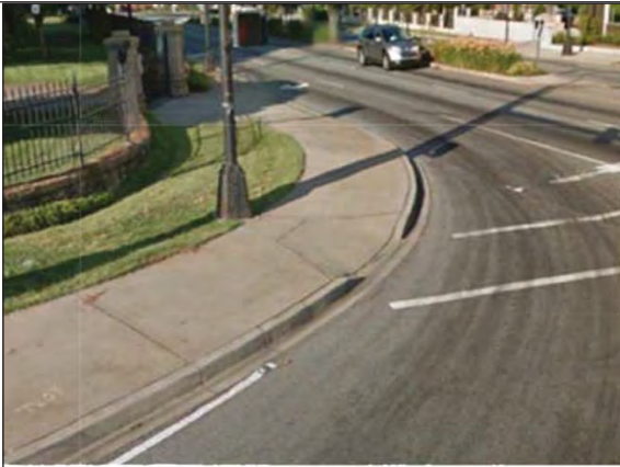
Sidewalk, Curb & Gutter, Existing Ramp
