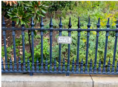
Fencing separating park area from the sidewalk
