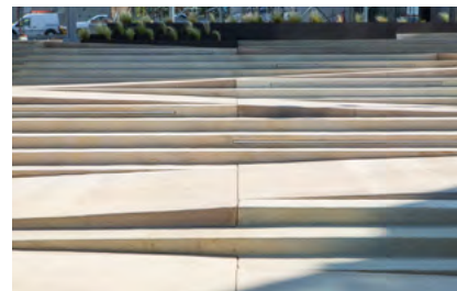
A "stramp" functions as both stairs and a ramp to provide accessibility, and can add stadium-like seating (The Boro Tysons)
