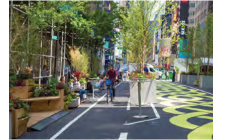
Roadway restriping to create more space for cyclists, pedestrians, and transit
