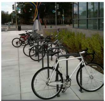
"Inverted-U" racks are an example of an acceptable rack design. These racks provide two points of contact, can secure a bicycle with a U-lock, and are securely anchored. They are also properly spaced from one another; and are located near the building entrance.
