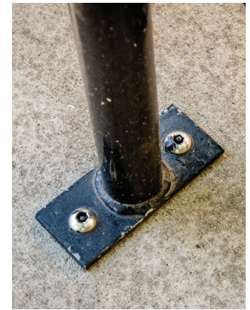
Flange (surface) mount and tamper resistant nuts
