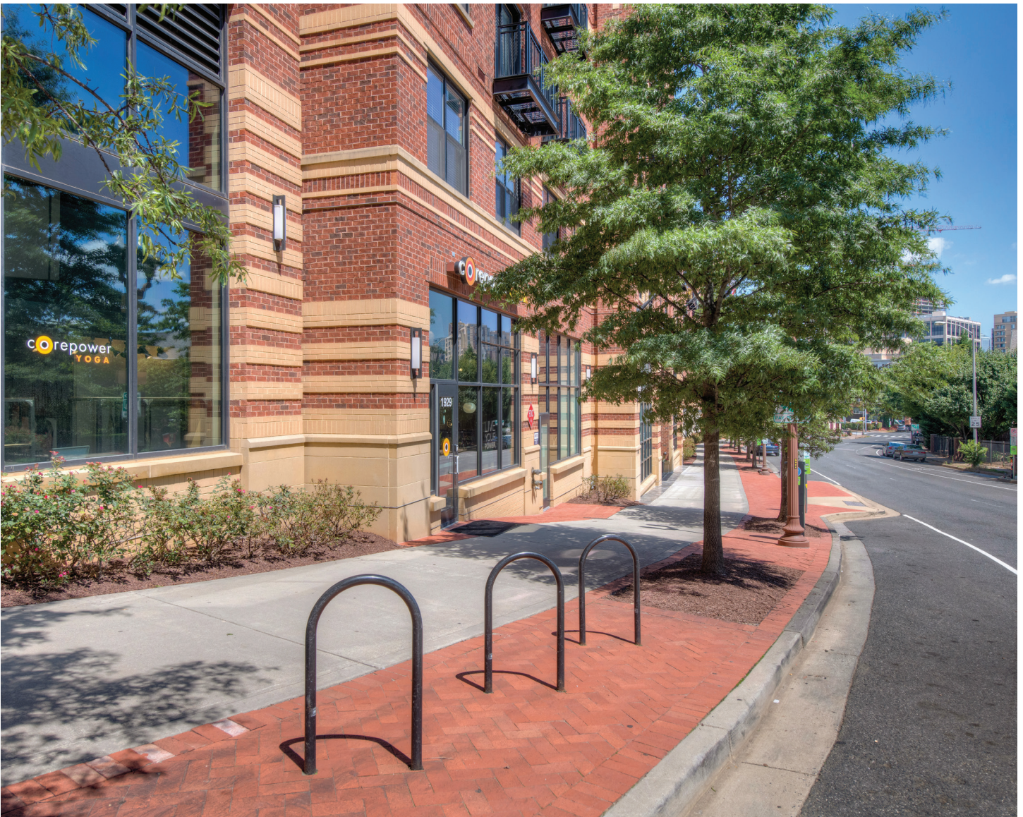
Sloped sidewalk installation
